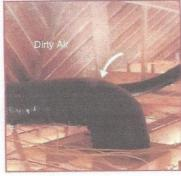
Sealing your ducts helps keep cleaner, filtered air inside while preventing sawdust, wood fibers, insulation particles, and unfiltered outdoor air from infiltrating your home.
